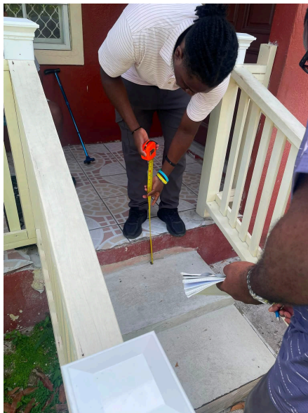
Special Projects 2: A Special Projects Unit team member takes measurements for accessibility improvements at a resident's home.
